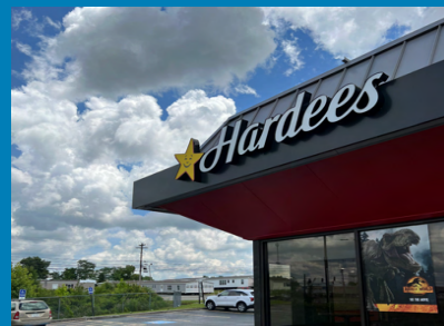
ACM Exterior Fascia
