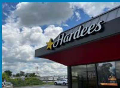
ACM Exterior Fascia
