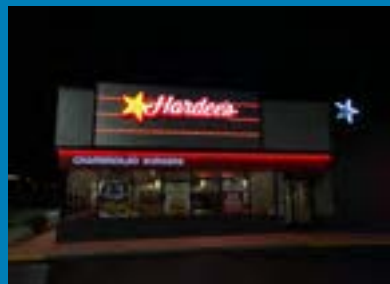
Cove Lighting and LED Retrofits
