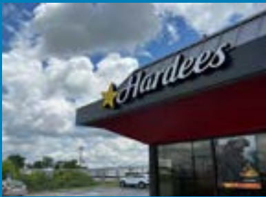
ACM Exterior Fascia
